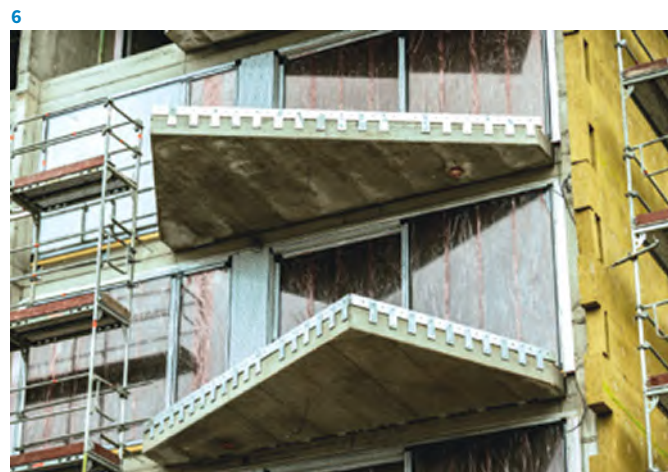
1 Situation 2 Visualisation 3 Sheet pile wall anchored in two levels by temporary anchor cables 4 Buildings of section A in September 2022 5 One of the buildings in section A with triangular balconies 6 Isokorb elements were used to break the thermal bridges
