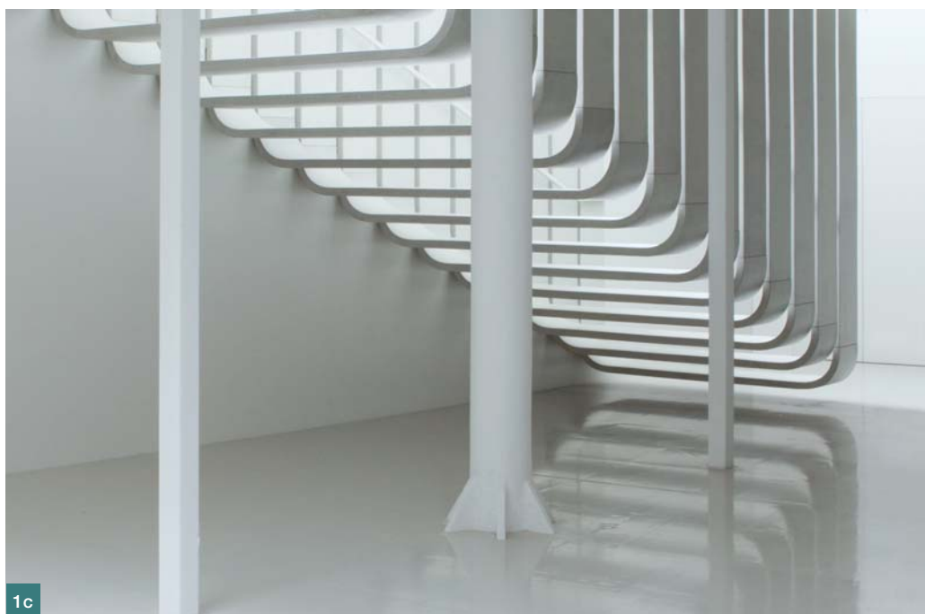
Obr. 1a-d Schodiště z UHPC ■ Fig 1a-d Staircase made of UHPC
