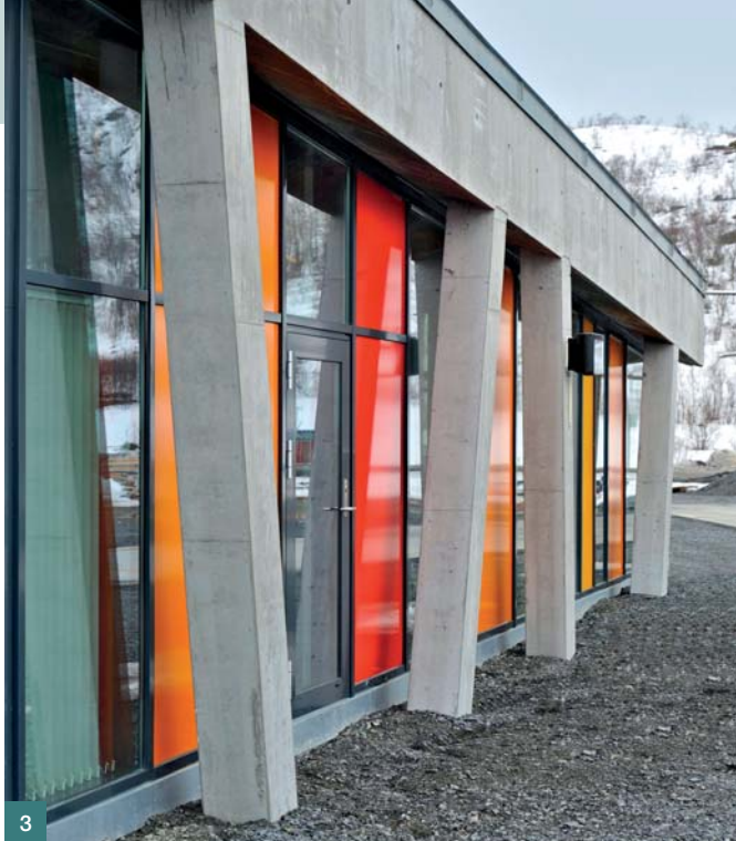
Obr. 3 Detail fasády ■ Fig. 3 Details of the facade
