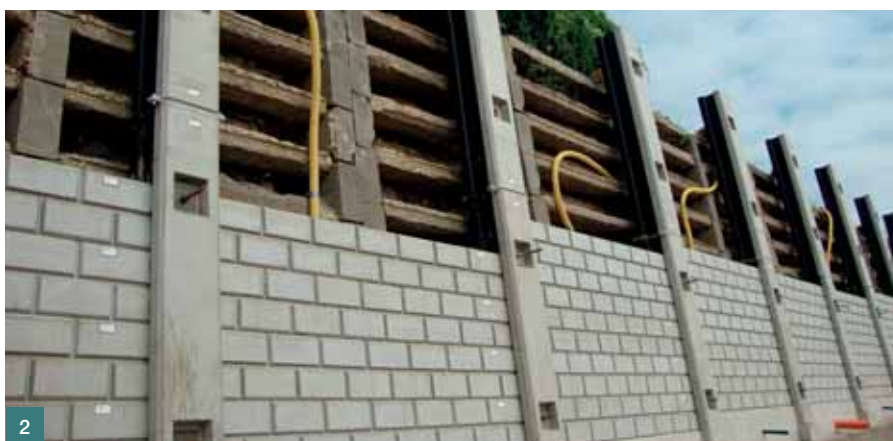
■ Fig. 2 Construction stage – gradual application of prefabricated surface elements
