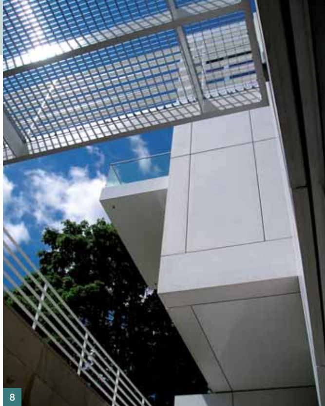
Obr. 5 Vjezd do objektu ■ Fig. 5 Entry in the building
