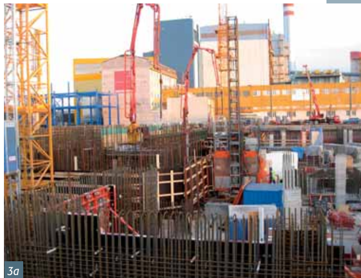
Fig. 3 Construction of stair towers, a), b)
