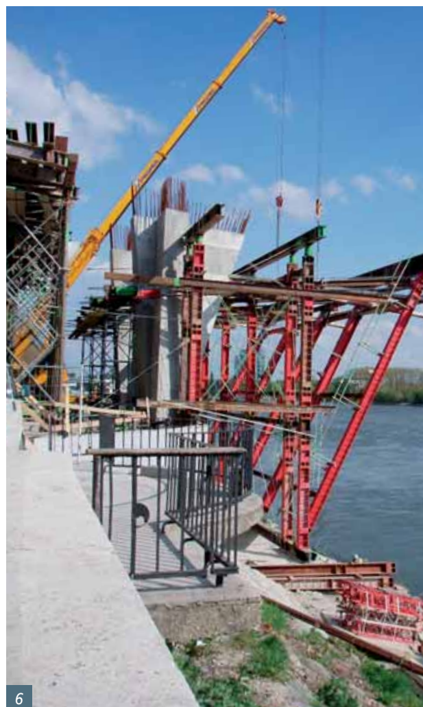
Fig. 6 Mounting of the shoring structure for cantilever above river
