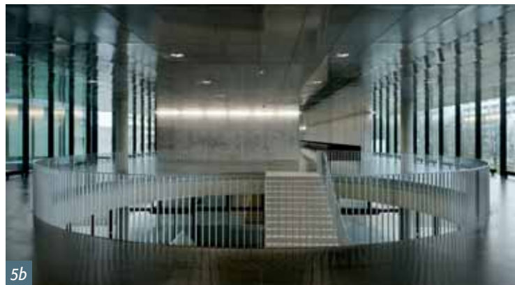
Fig. 5 Faculty of Chemical Technology – a) central staircase, b) entrance hall in the 2nd floor, c) core of the lift in the hall with a clear graphic marking, d) marked stand-alone ramp leading into the entrance hall on the 2nd above-the-ground storey
