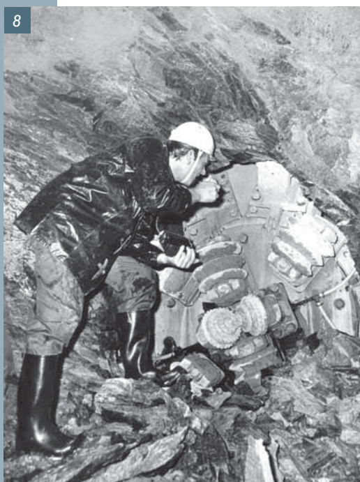
Fig. 12 Part heading shield machine RŠF-1 with a road header
