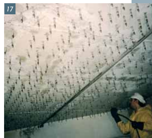
Fig. 17 Injection of the grid of the ceiling of the underground garage
