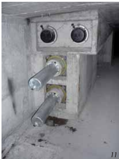
Fig. 12 Expansion joint
