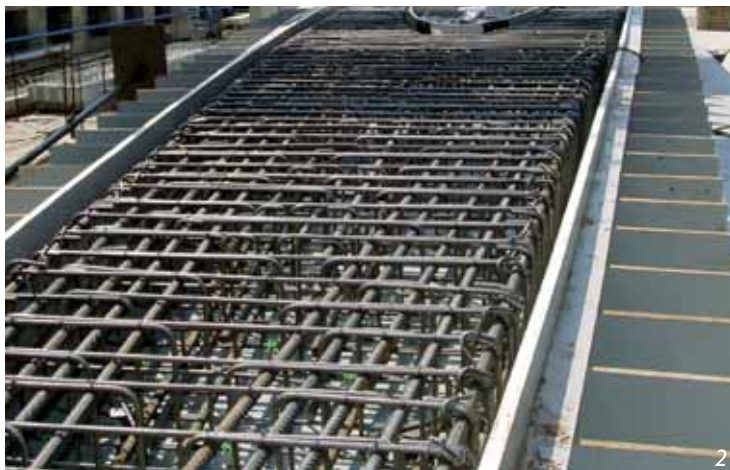
Fig. 3 Concreting a prefabricated part
