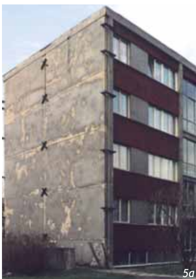
Fig. 2 Diagram of the deformation of gable panels HK-60
