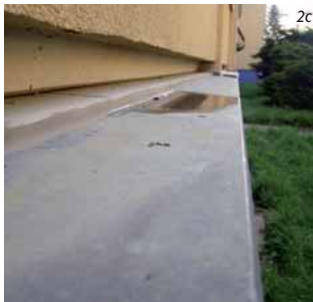
Fig. 2 Condition of the construction two years after the application of heat insulation of the external skin: a) view of the facade, b) detail of the balcony with visible continuation of corrosion of the reinforcement; impact of temperature movements of corrosion products on concrete cohesion, c) downgrading of balcony plating with possible water leakage into the balcony structure, d) proof that the cracks between the panels of the external skin are alive – pattern of the cracks in the newly applied facade
