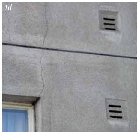
Fig. 1 Prior to applying thermal insulation: a) view of the facade, b) detail of the external skin with visible corrosion of the reinforcement accompanied by „blasting“ of covering layers of concrete, c) an unsuitable original detail of the sheeting which allows water to leak in the structure of the balcony, d) cracks in places where the external panel is weakened by the window opening
