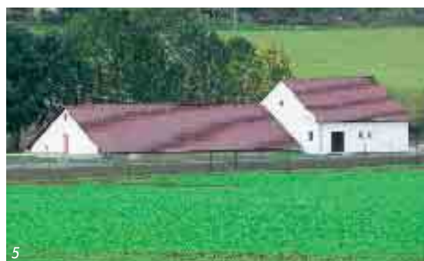
Fig. 5 Wastewater treatment plant Buštěhrad – general view
