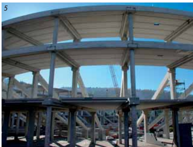
Fig. 6 Placement of bended spandrel beams – general view
