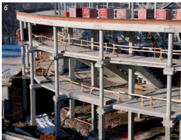
Fig. 6 Placement of bended spandrel beams – general view
