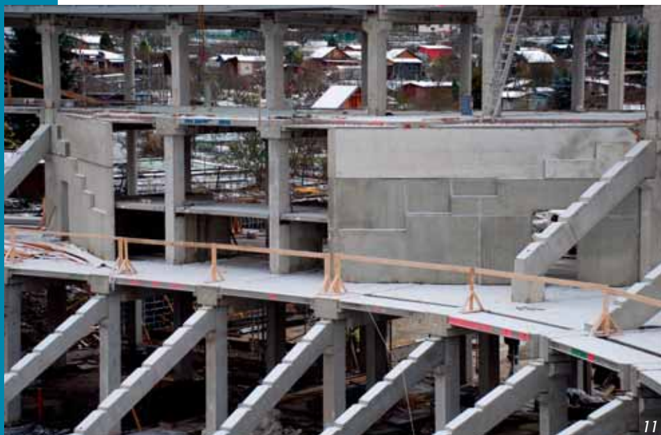
Fig. 9 Atypical corner – coupling of radially arranged girders to the orthogonal system – frog's eye perspective
