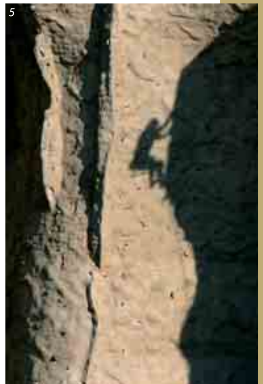
Fig. 5 Detail of the wall
