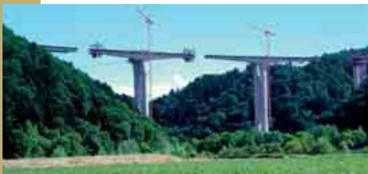
Fig. 1 Cantilever construction of frame prestressed bridges – Pont sur La Mentue
