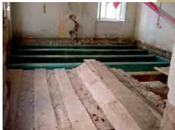
Fig. 6 Reinforcement of roof slab of street bay
