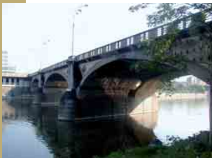
Fig. 1 View of the upstream side of the bridge
