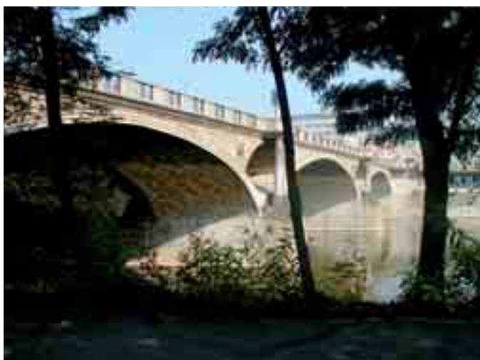
Fig. 2 View of the downstream side of the bridge
