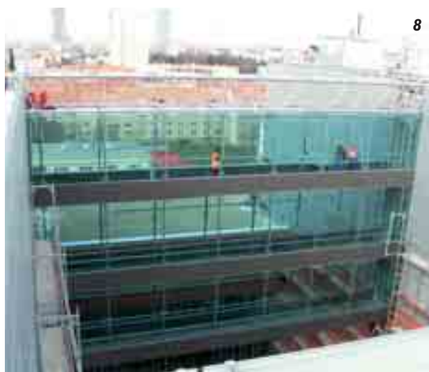
Fig. 10 Placing of truss girder on concrete attic
