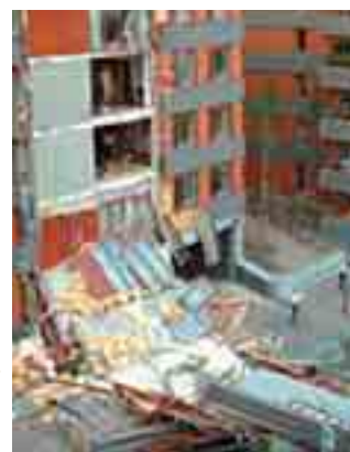
Fig. 11 Progressive collapse of a series of balconies, Maastricht, The Netherlands, 2003
