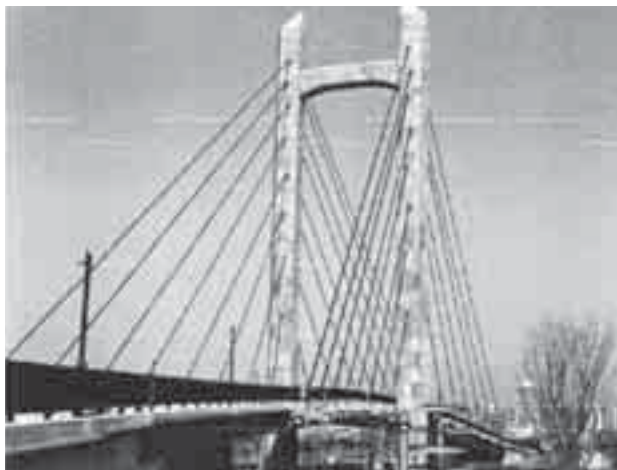
Fig. 29 Shin-kiba Ohashi bridge
