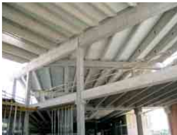
Fig. 9 Main entrance space adjoined to the storey
