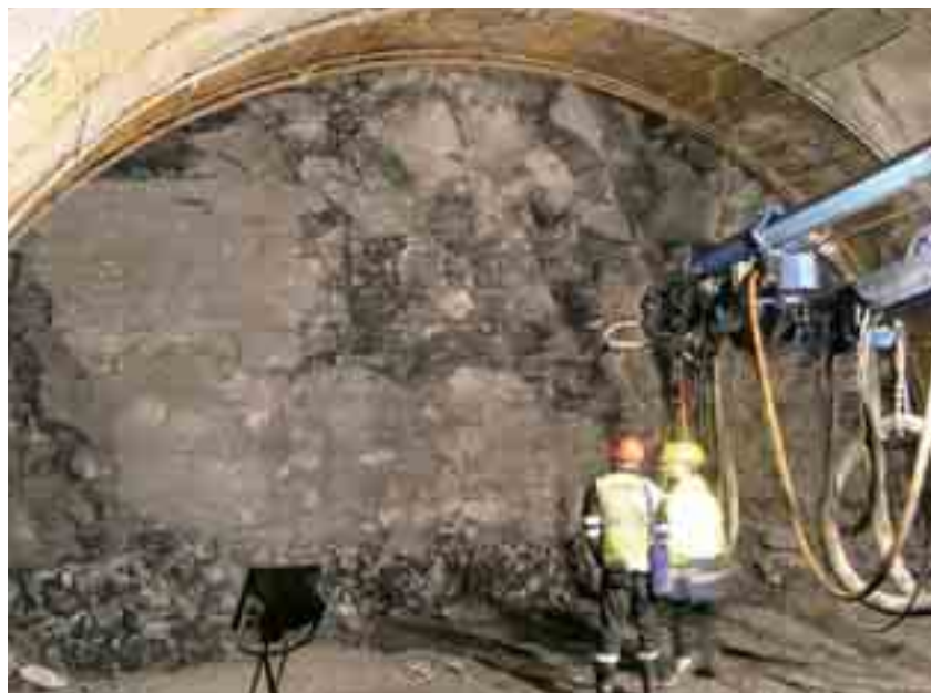
Fig. 6 Face of the tunnelling and primary lining
