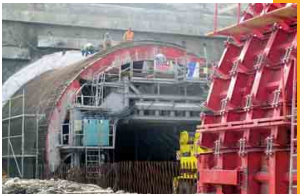
Obr. 2 Samonosná ocelová forma Fig. 2 Self-supporting steel mould
