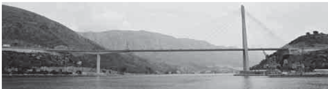
Fig. 30 A view of the completed Dubrovnik bridge
