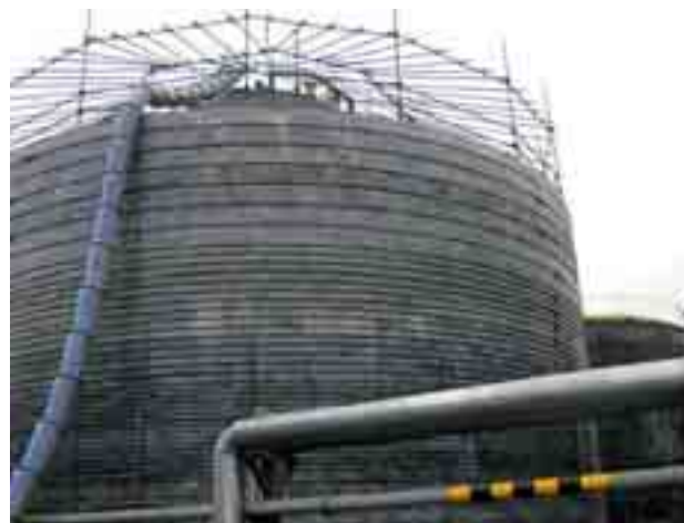
Fig. 3 Maintained reservoir before construction of outer surface
