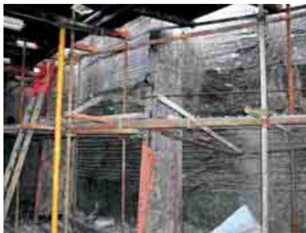
Fig. 2 State of patent wire braid after removal of outer surface
