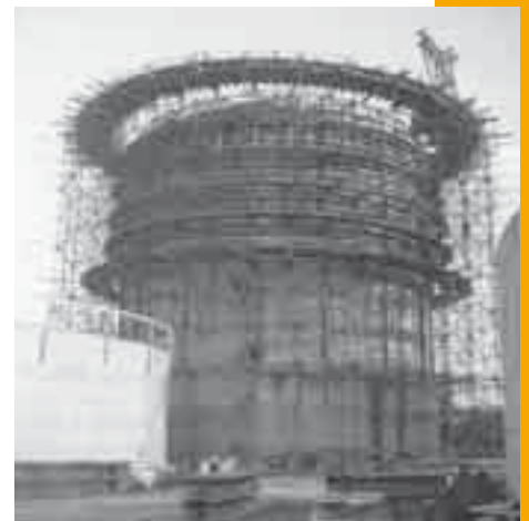
Fig. 3 The tank after concreting of the upper part with scaffolding and formwork
