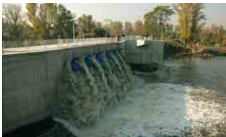
Fig. 13 Operational test of the pumping station
