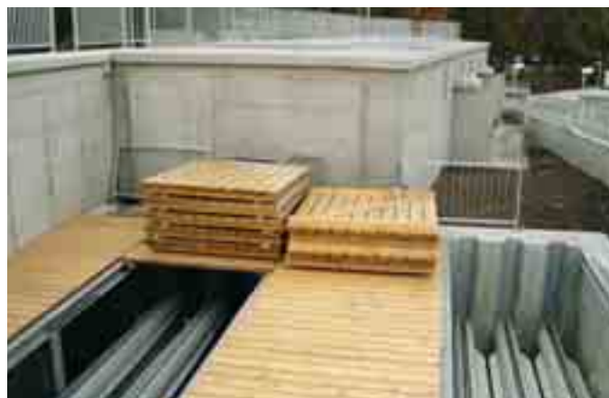
Fig. 4 Finished pumping station and a storage of stoplogs
