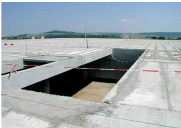
Fig. 11 View of the floor structure with openings for escalators
