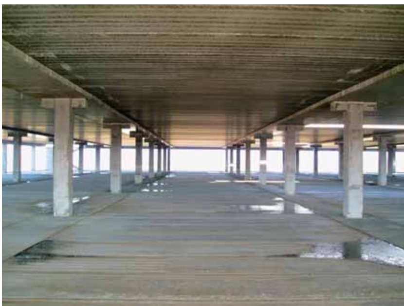
Fig. 17 View of the internal structure of the prefabricated construction
