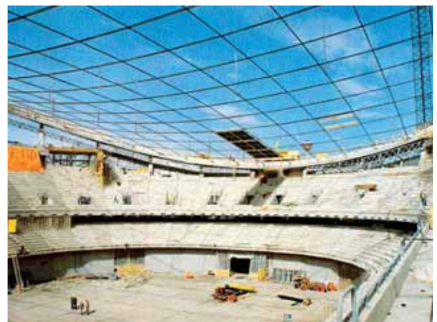
Fig. 48 Olympic stadium "Saddledome", Calgary – erection of the roof
