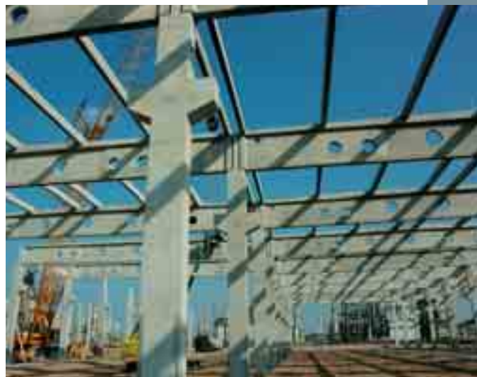
Fig. 10 Paper-mill Leuna under construction
