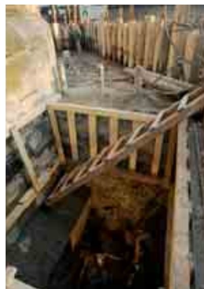
Fig. 5 An exploration well by the pier no. 8
