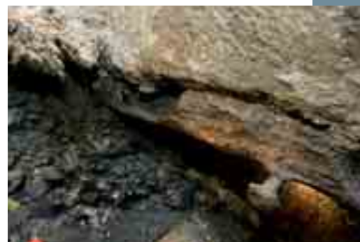
Fig. 7 A detail of an iron bolt protruding from a beam under a set-off foundations
