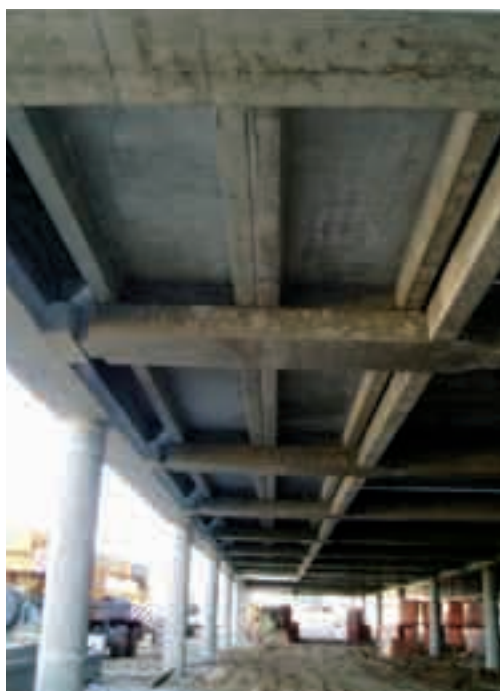
Obr. 8 Podhled na strukturu stropu s travelátory Fig. 8 Ceiling for the floor structure with travellers
