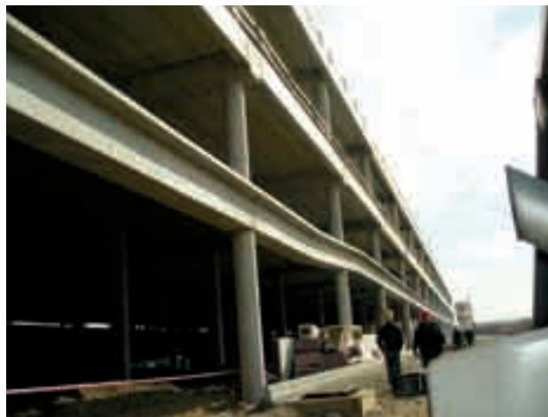
Fig. 12 Peripheral supporting structures for the steel structure placement in the arrival hall
