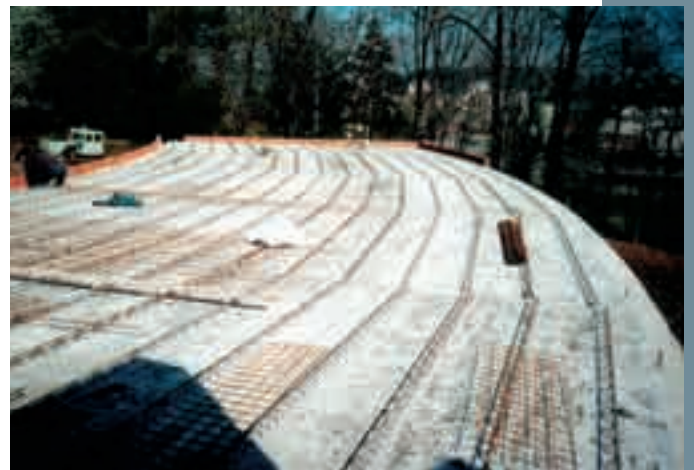
Fig. 6 Structure of filigrane units, part "B"
