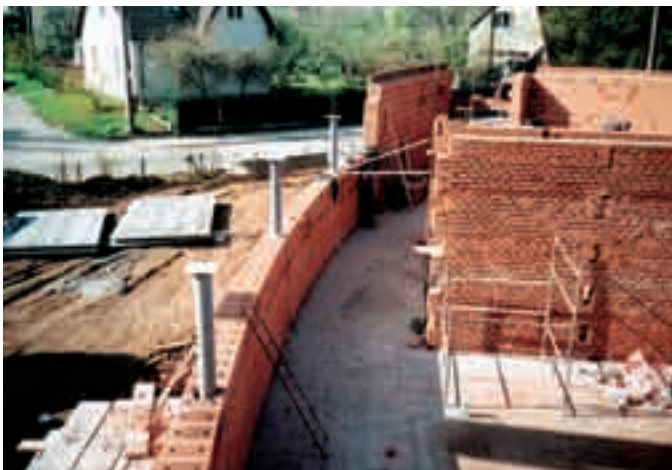
Fig. 5 Brickwork and mounting of steel columns of residential part "B"
