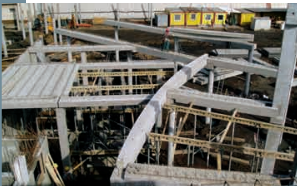
Fig. 11 Benches and entries with a bearing floor structure built from PARTEK panels
