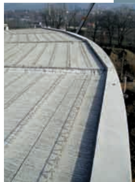
Fig. 8 Ceiling with filigranes and a covered peripheral supporting structure
