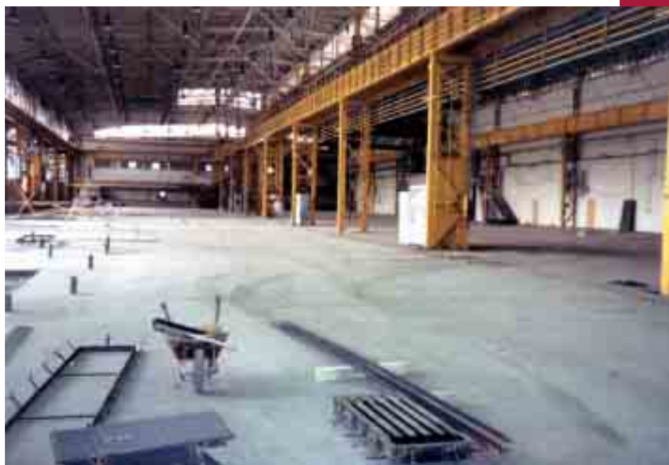
Fig. 1 Concrete floor of the production hall under reconstruction
