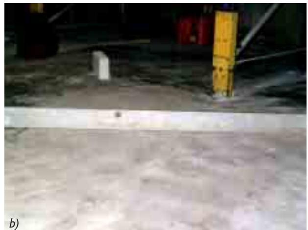
Fig. 6 a) manual regrinding of the repair surface, b) the final condition after removal of excessive sand, roughness below the lath not exceeding 1 mm
