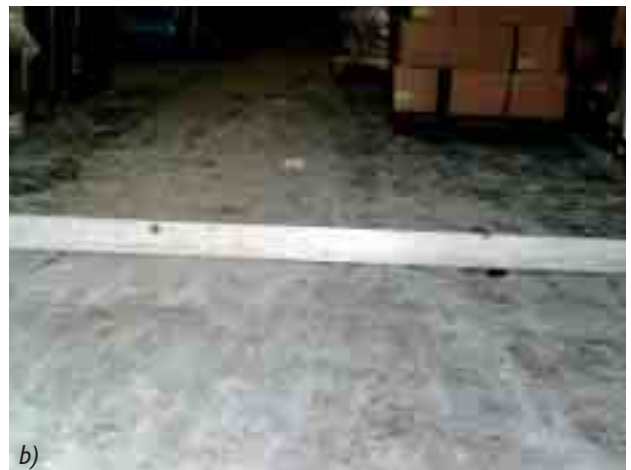
Fig. 3 a) local unevenness in the “repaired” storeroom floor, joint in front of the carriage, b) sinkage in the transverse direction to the passage between the storage racks
