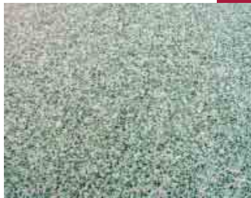
Fig. 8 Epoxide floor with multicoloured silicic sands
