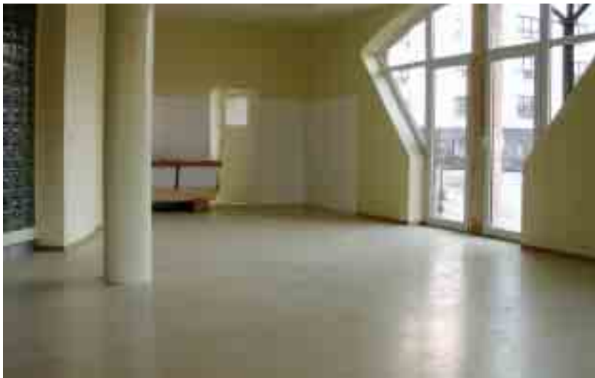
Fig. 7 Epoxide floor in a health centre
