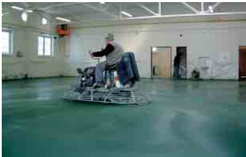
Fig. 4 Finishing floors with a two-disk and edging floor grinder
