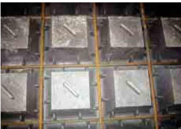
Fig. 6 View of main reinforcement placed on distance ribs
