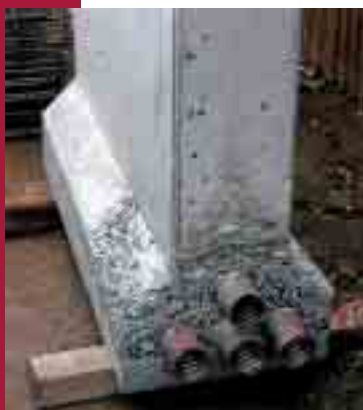
Fig. 9 First – not perfectly concreted experimental section
