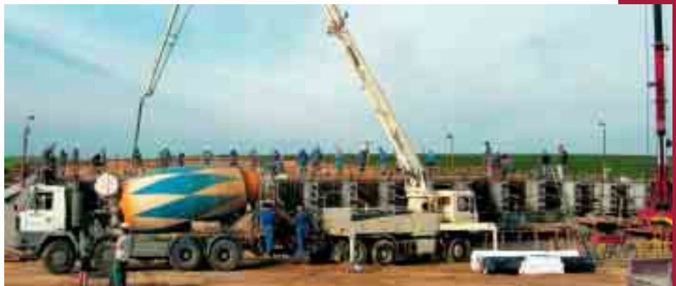
Fig. 12 Concreting in the whole breath of the slab needs larger crew
