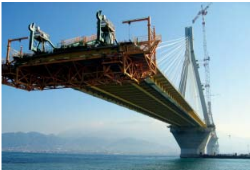
Fig. 3 Completion of the first cantilever in November 2003
