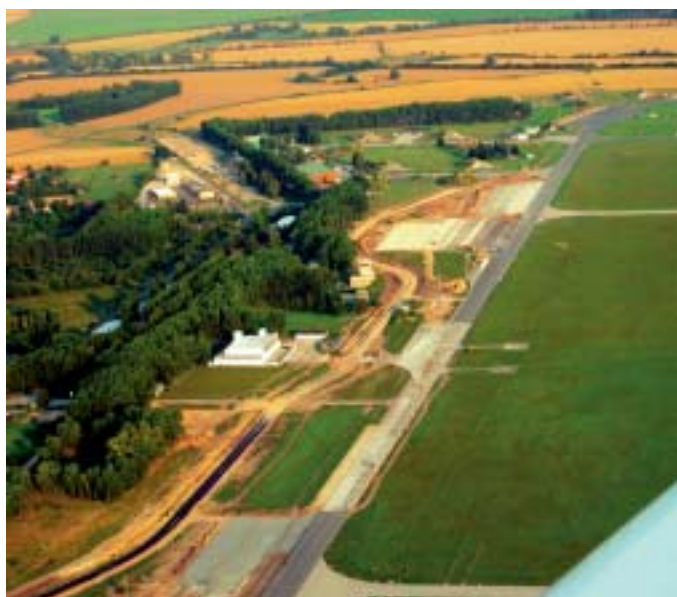
Fig. 4 An aerial view of the construction of the AB Čáslav
