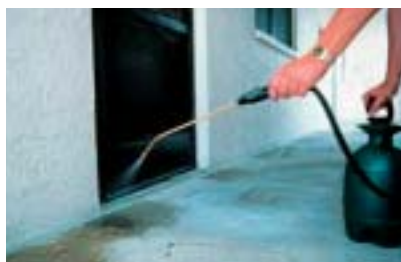
Fig. 5 Easy application of the Protectosil CIT preparation
