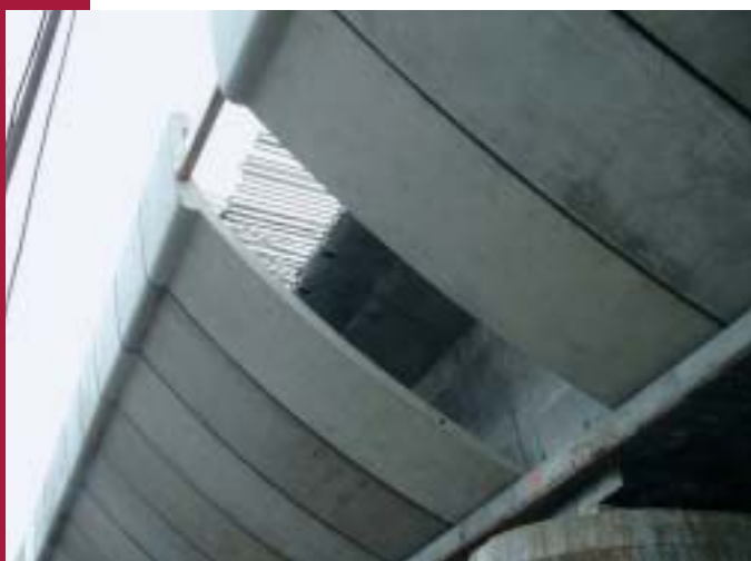
Fig. 1 The shape and composition of prefabricated struts on the bridge structure
