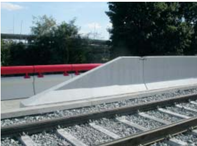
Fig. 5 An untypical safety fence, creating a separating wall
