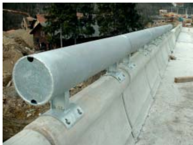
Fig. 3 The upper part of the strut with a mounted steel handrail
