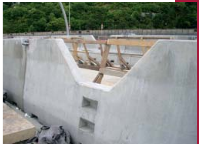
Fig. 6 A passage opening in the prefabricated wall
