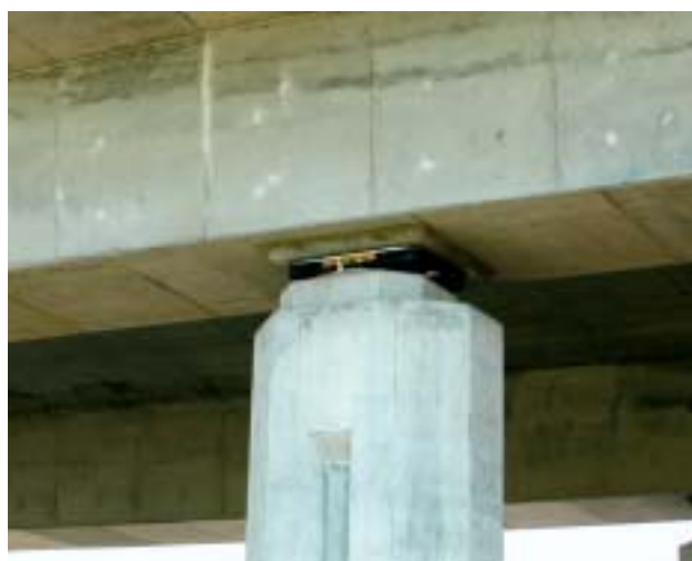
Fig. 11 Detail of the bridge bearing of the elevated road
