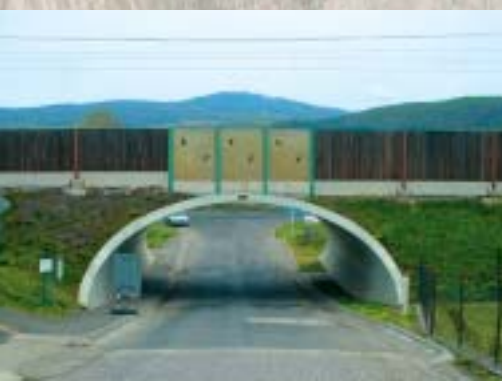
Železniční most v km 502,155 trati Lovosice – Ústí nad Labem Railway bridge, km 502.155 on the railway route Lovosice – Ústí nad Labem
