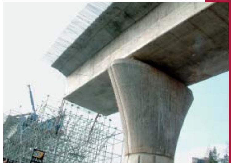
Obr. 6 Estakáda Hlubočepy-Barrandov, detail Fig. 6 Elevated road Hlubočepy-Barrandov, the detail
