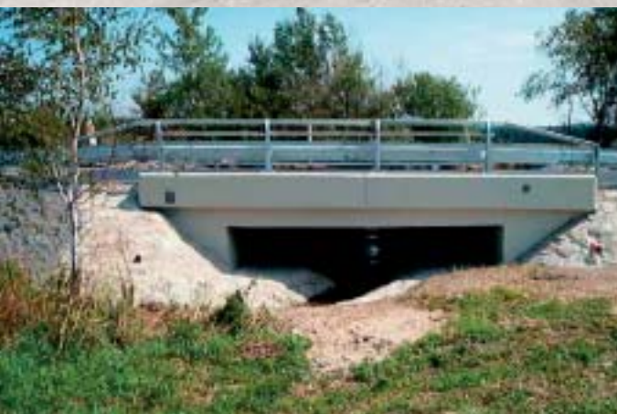
Oprava mostu na silnici I/21 Bridge repairs on I/21 road
