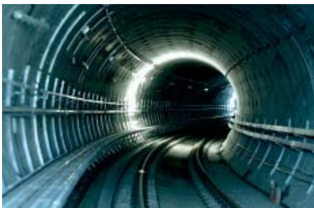
Fig. 7 Great Belt Link, east tunnel, Denmark, design life 100 years
