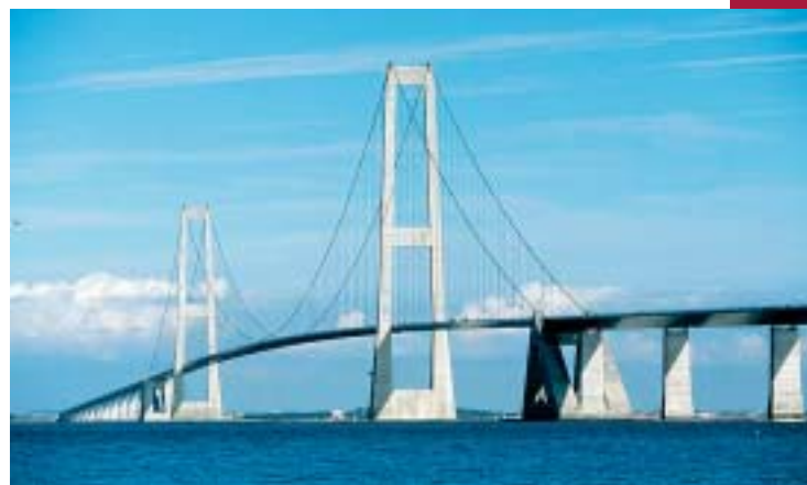
Fig. 8 Great Belt Link, east bridge, Denmark, L = 1416 m, design life 100 years
