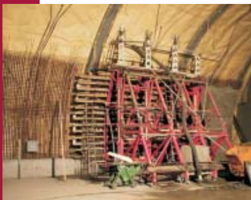
Fig. 6 Concreting of the vault side
