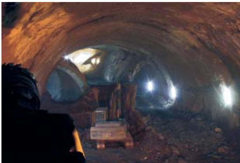
Obr. 2 Ražby rozpletu Fig. 2 Driving of the tunnel branching
